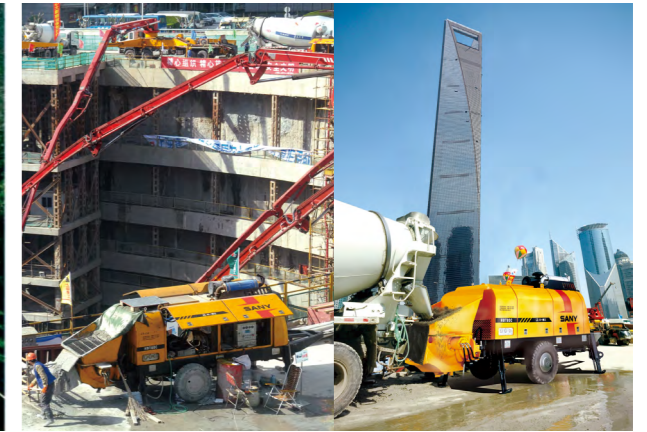
SANY Trailer-mounted Concrete Pump's Construction at Shanghai Tower.
