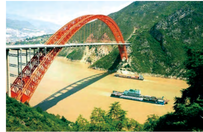
SANY Trailer-mounted Concrete Pump's Construction in Wushan Yangtze River Bridge Project
